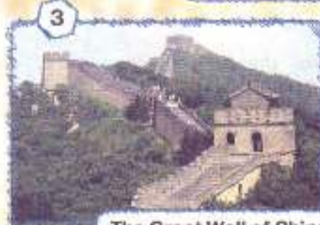
The Great Wall of China
